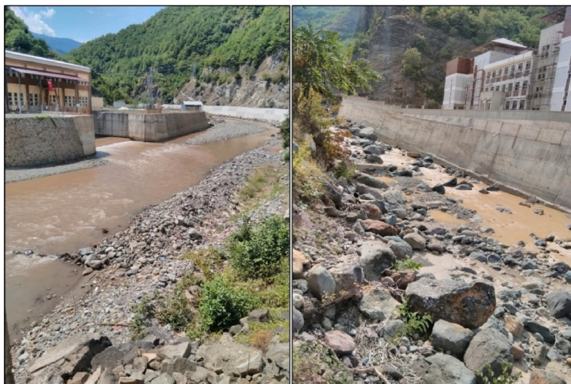
Fig. 14. The common application of constructing concrete walls along the streambed to stabilize the banks to protect both the roads and RoR-HEPP facilities (on the left), and houses/buildings (on the right) in the lower part of the Murgul Stream.
