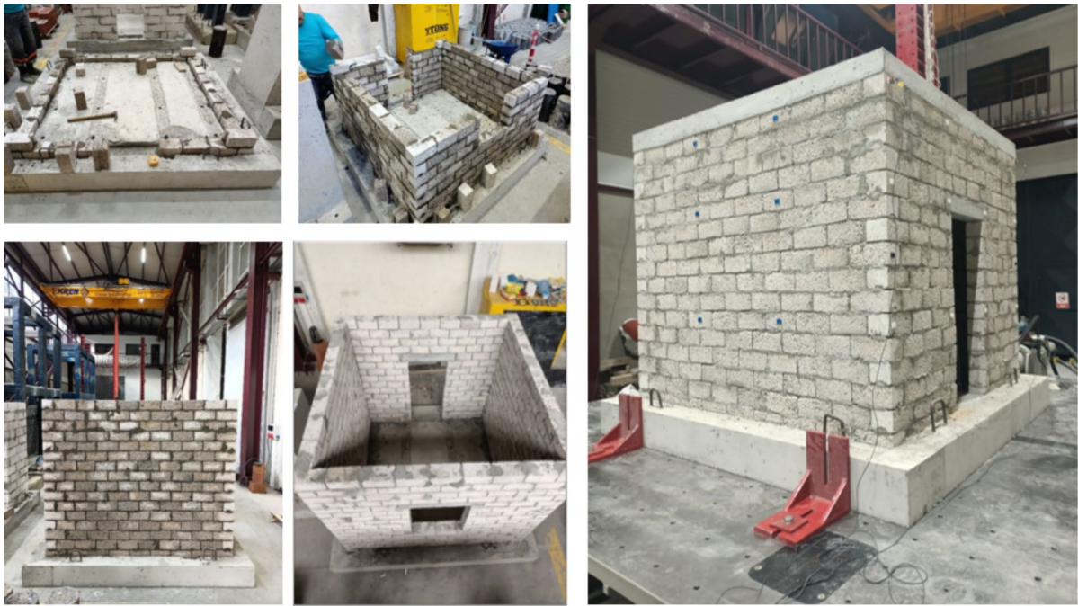
Fig. 3 Images of pumice wall construction stages
