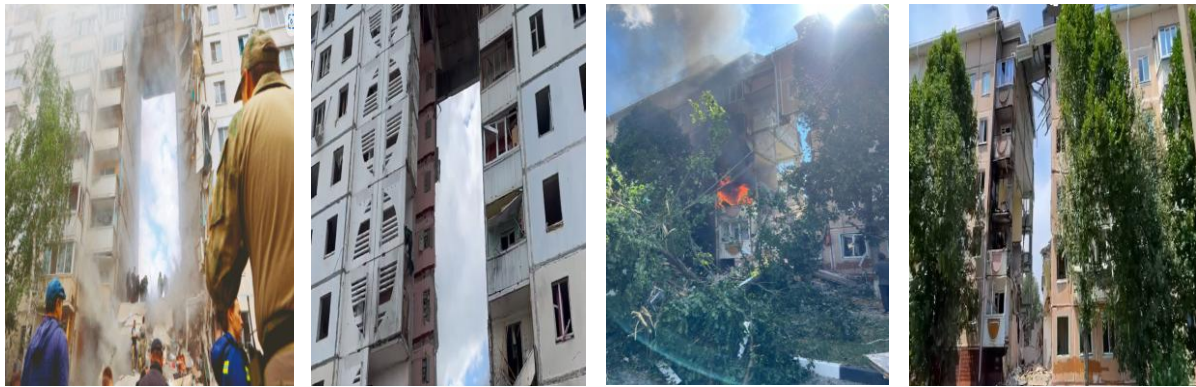
Figure 13. Examples of Progressive Collapse (Governor of Belgorod, 2024).
