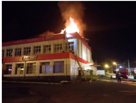
Figure 14. Damage to the structure caused by FVP (Governor of Belgorod, 2024).
