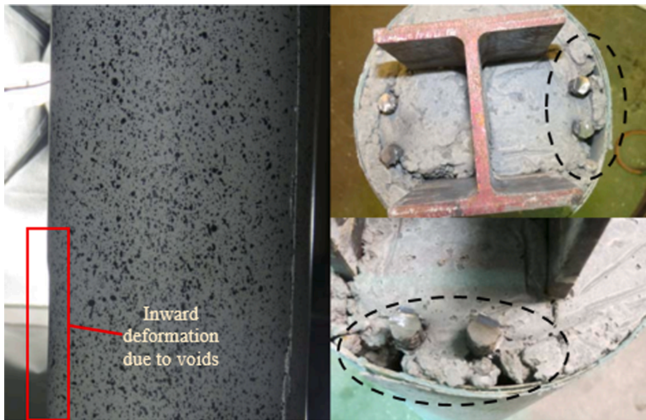
Fig. 16. Construction error during concrete casting of G4/2/4#4.
